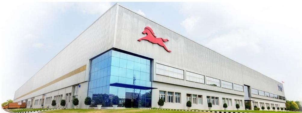
TVS Motors Plant-2
