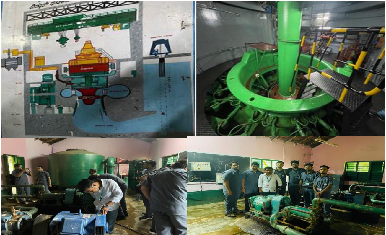
Linganamakki Power House, Sagara Taluk - Photos
